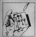
1. Rewire the tagged wires to their respective terminals on replacement operator.
