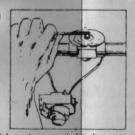
2. Valve stem must be in open position when replacing deperator. Stem is in open position when stem slot is in line with pipe run. It stem slot indicates closed position insert screwdriver in slot and turn until slot is in line with pipe run. Never attempt to turn the motor actuator on the operator as this would damage the motor.
